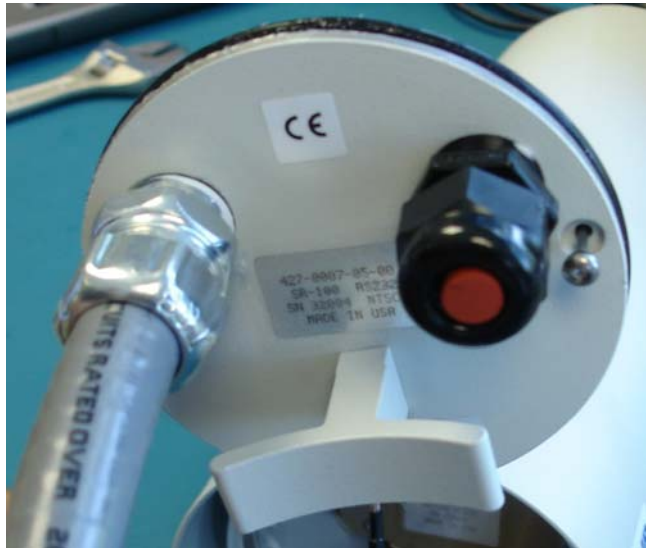
Figure 4: Cable Gland Plug Installed
